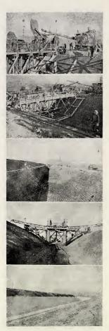
CONCRETING EQUIPMENT, CANAL SECTION. REINFORCING STEEL PLACED IN CANAL. CANAL TRIMMER. LINED CANAL.
